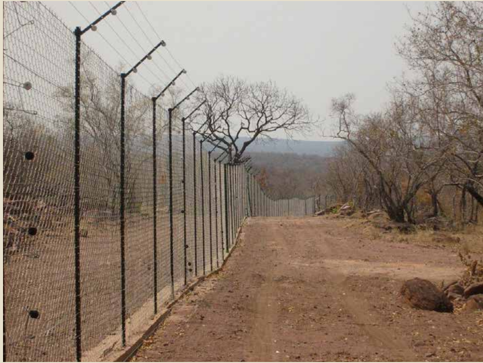
Figure 41: Leopard-proof fencing used around herbivore enclosures in Maharashtra, height of fences is usually more than 12feet above ground and 1 feet below ground
